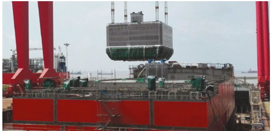
Installation of one of the two IHI-SPB tanks manufactured in Japan for the floating storage and regasification barge that Wison Offshore Marine built for Exmar
