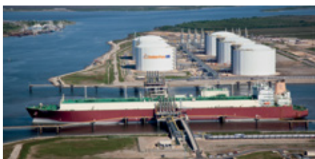
Built initially as an LNG import terminal, Golden Pass is to be provided with three 5.2 mta liquefaction trains
